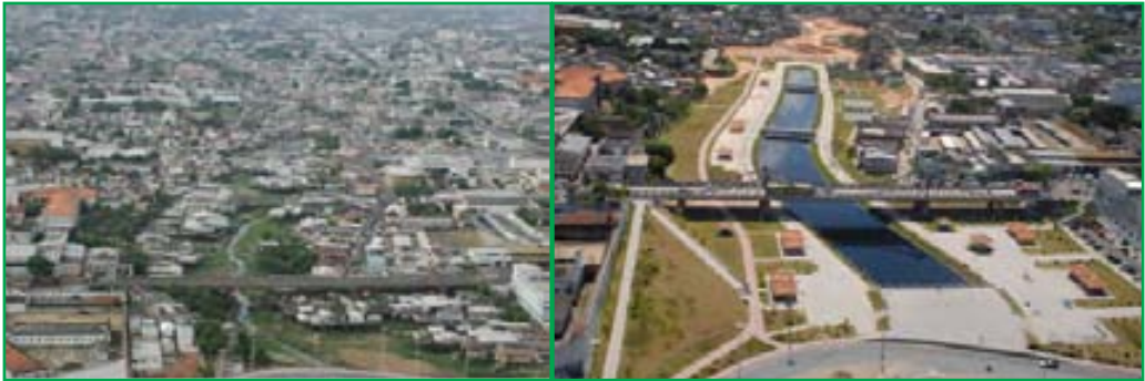
Figuur 4.14: Before and after pictures of the area around the Benjamin Constant bridge
